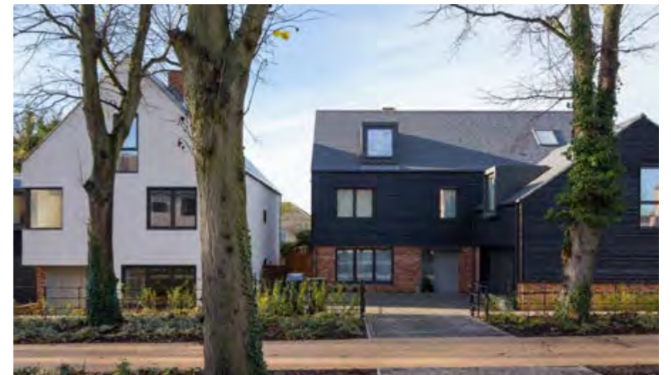
Above: Contemporary interpretation of larger family housing. Roof form creates variety within the street scene.
