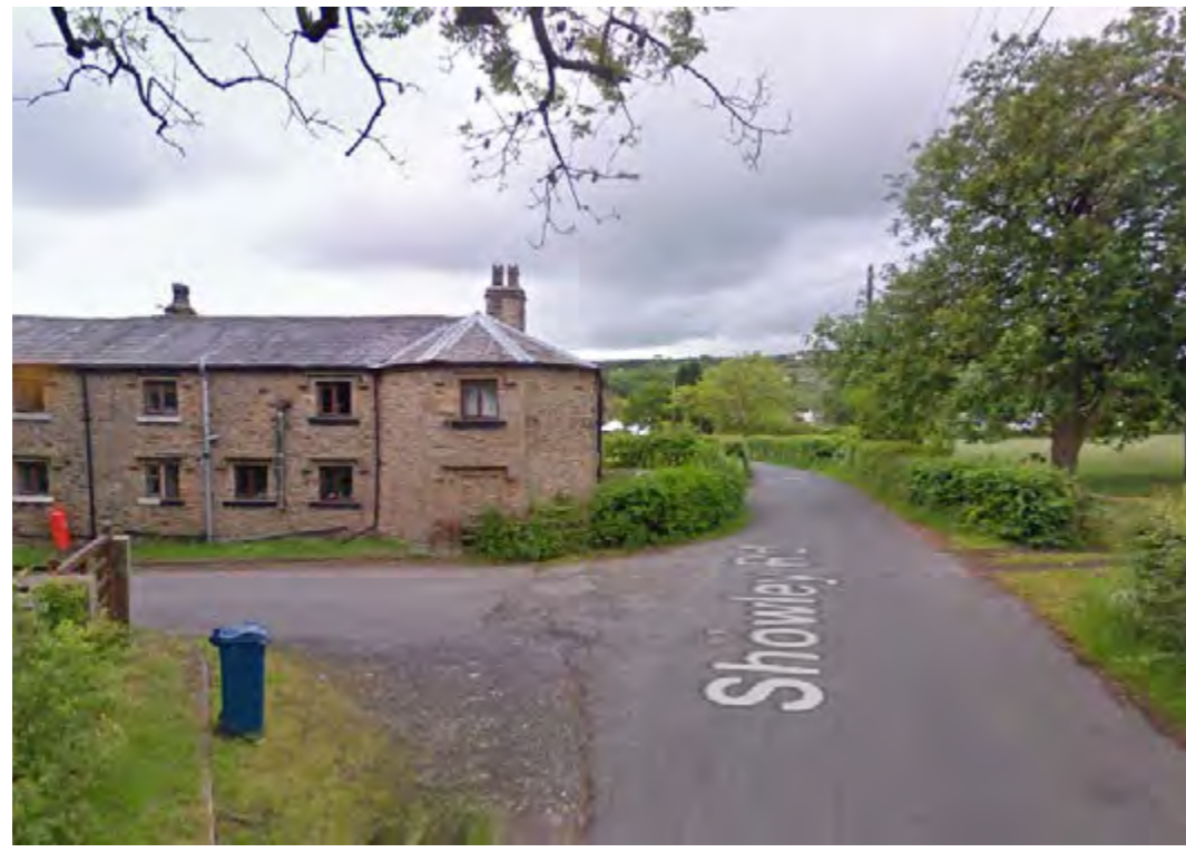
A CORNER BUILDING MARKS THE ENTRANCE TO THE FARMSTEAD AT THE JUNCTION WITH THE RURAL LANE
